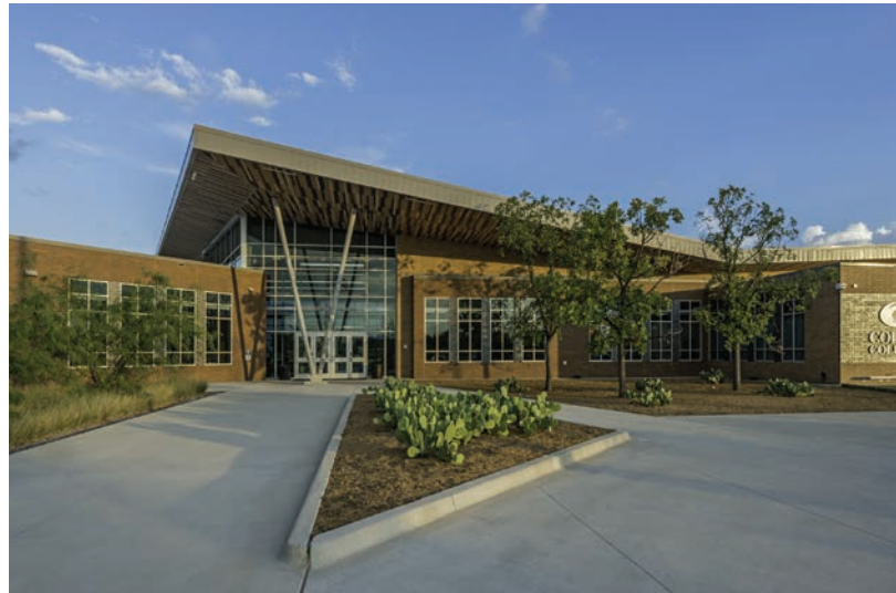
Collin College Public Safety Building
